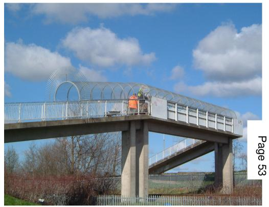
Photos 1 & 2: Enclosure Installed at Hough Green Railway Footbridge
